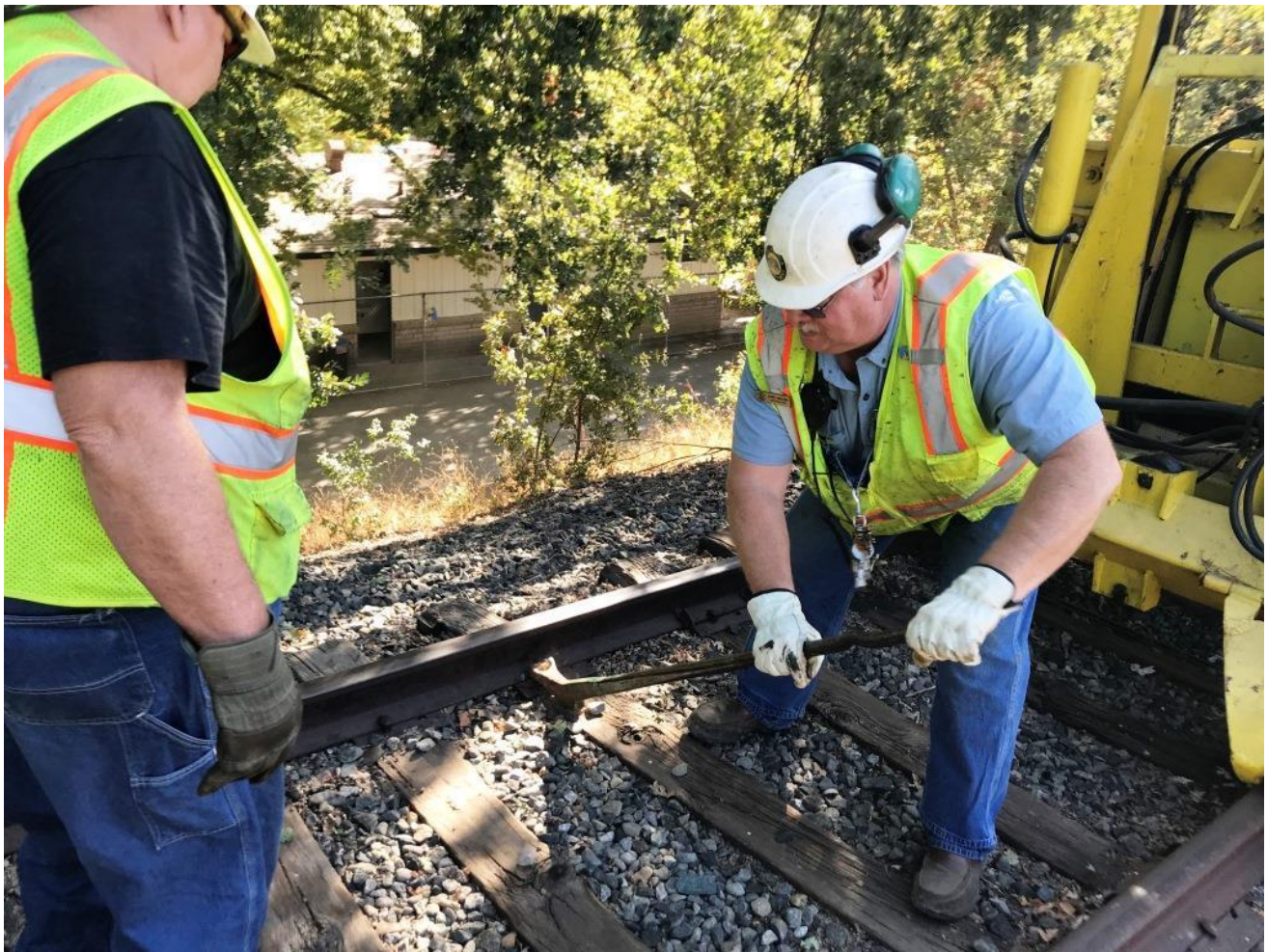
Chris and Harry pull spikes on a tie slated for removal
