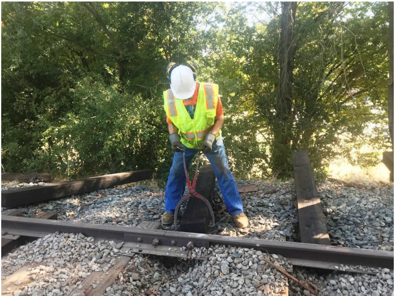
Clem gets a tie lined up for the scarifier to pull in
