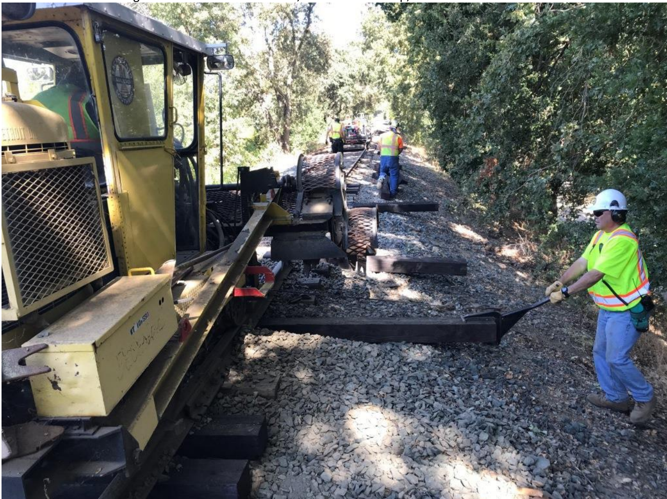
Taka now works with the scarifier-inserter to pull in another new tie
