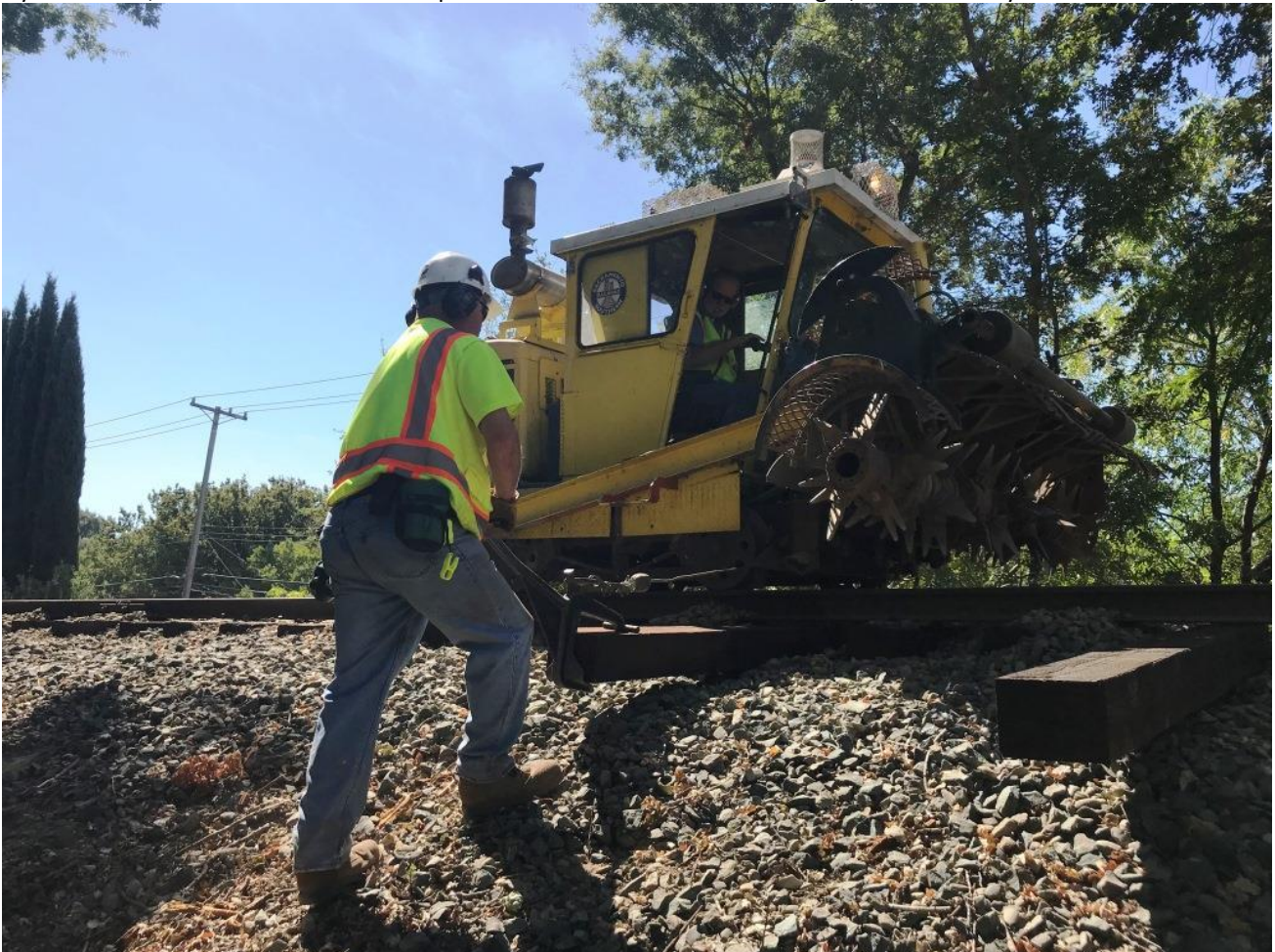
Taka guides a new tie as Alan in the scarifier pulls it under the rails
