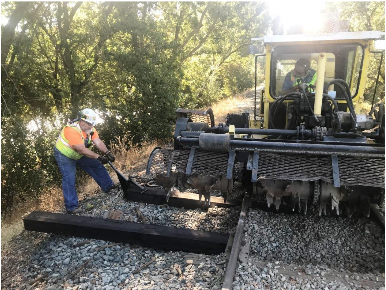
Alan brings in the scarifier-inserter and, with Mike F.'s help, inserts a new tie under the rails
