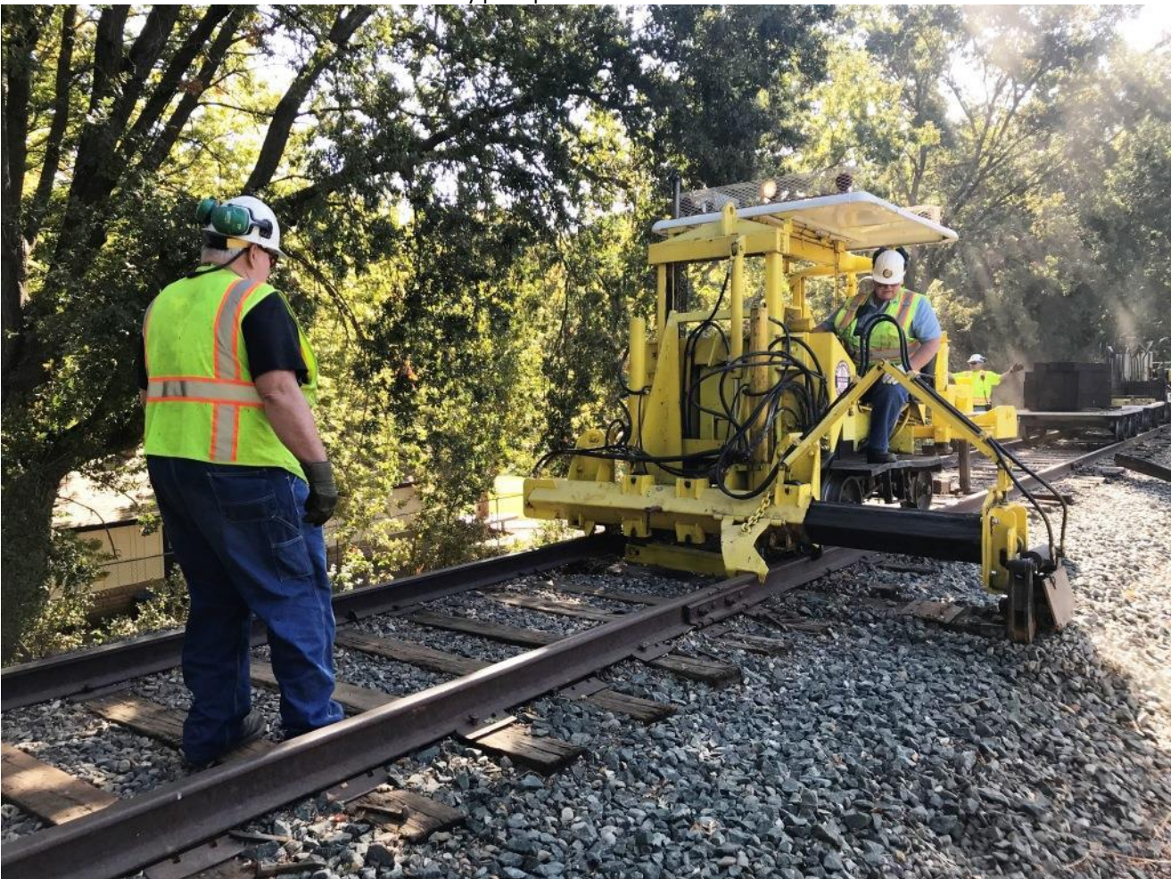
Chris on the 125 slides an old, rotten tie out from under the rails
