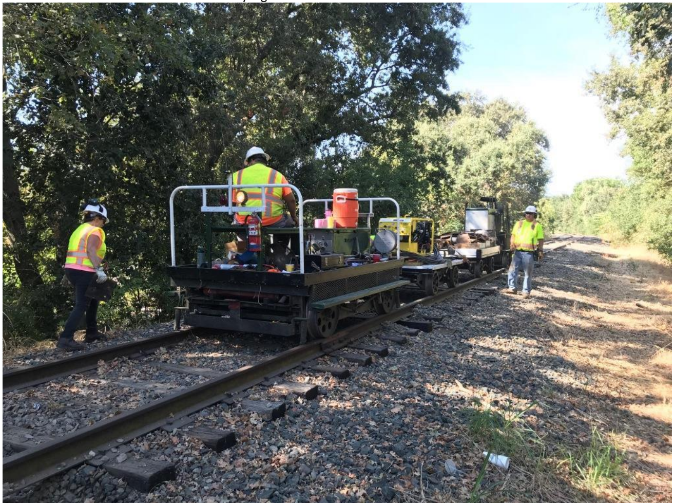
The Team does a sweep of the line to locate any tie-plates that may be lying about
