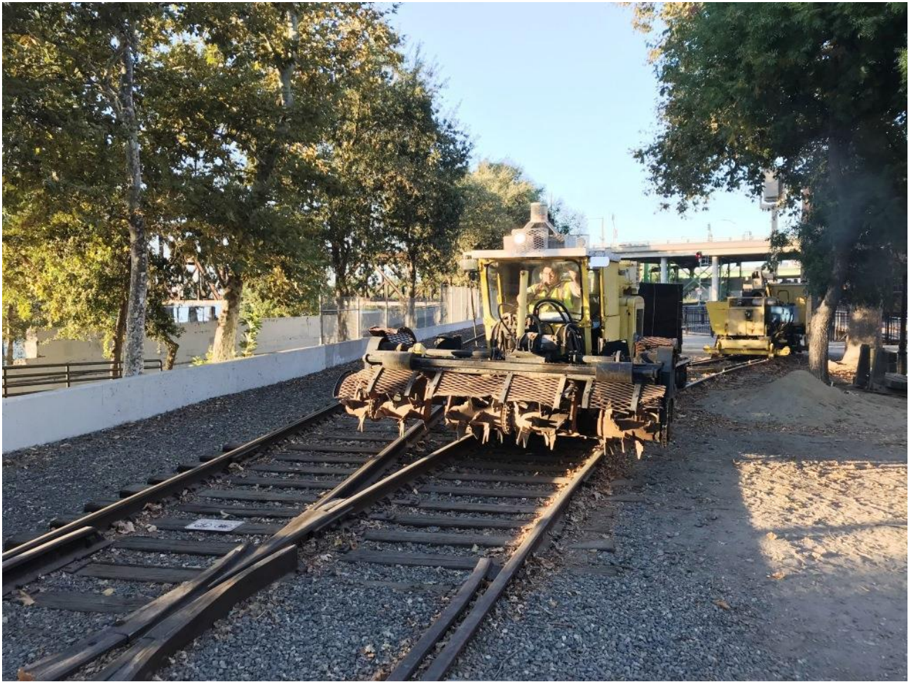
Anthony moves the scarifier off the North Turntable Lead
