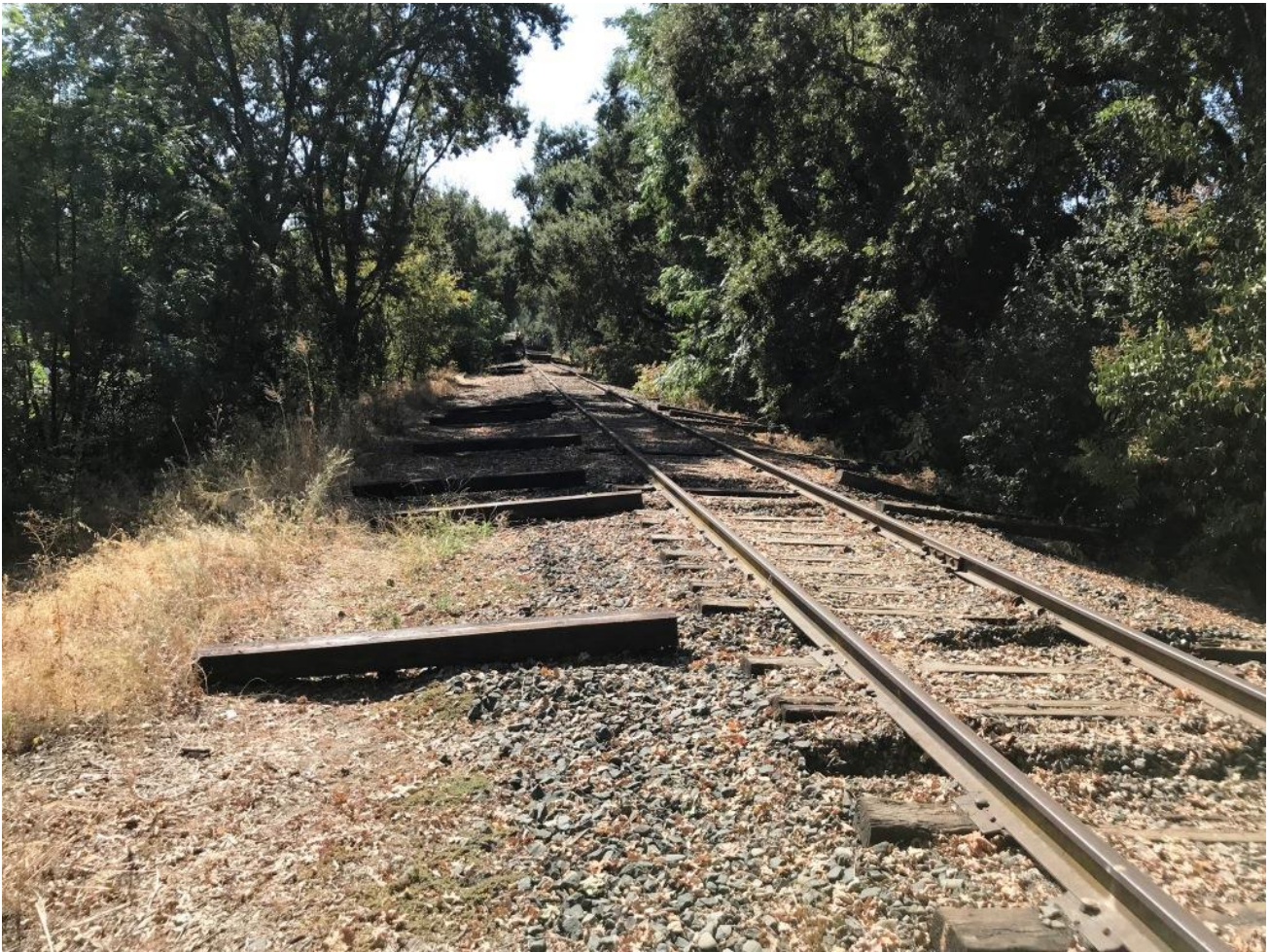
By lunch time, evidence of our work was plentiful: removed ties are on the right, new ties ready to insert are on the left
